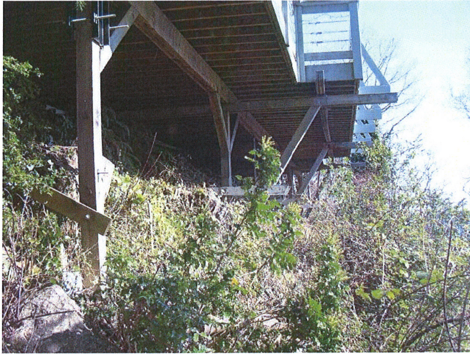
Photo 5. Looking east at vegetation beneath and below deck.
