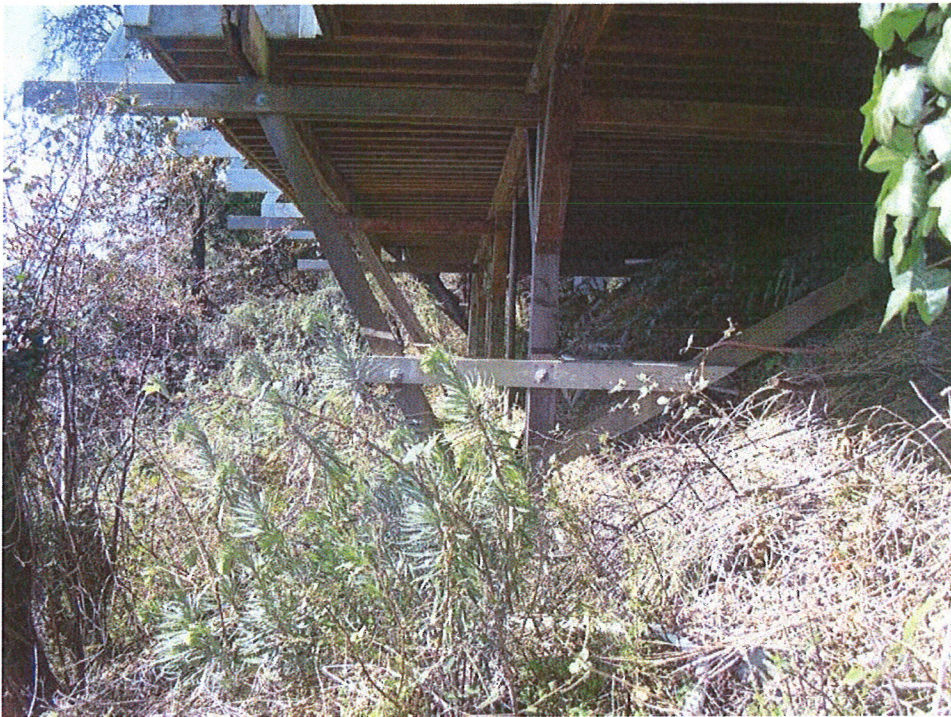
Photo 6. Looking west at vegetation beneath and below deck.
