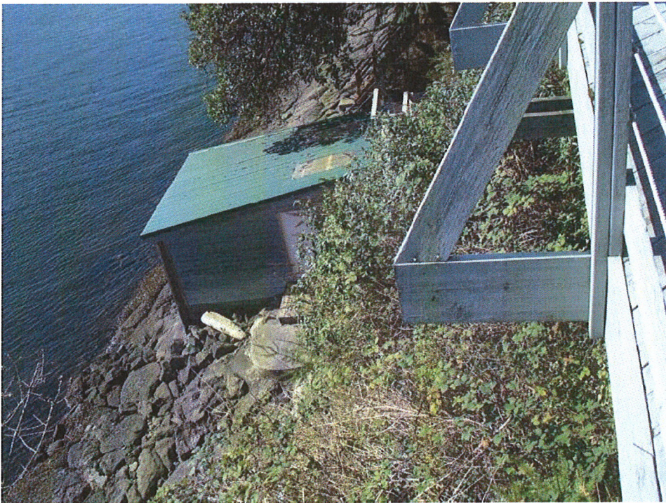
Photo 4. Looking west at vegetation below deck, beach and boathouse.
